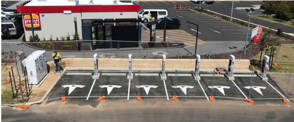
Fig. 2.7 Western Australia's first Tesla Supercharger site near Bunbury (photo: Tesla Owners Club WA, TOCWA)
