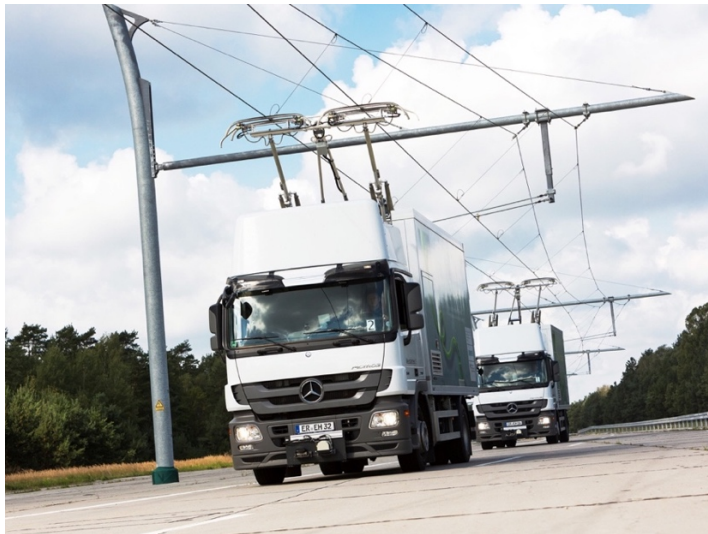
Fig. 1.13 Overhead power rails for electric trucks, (photo Siemens/Daimler-Benz [Wired 2017])
