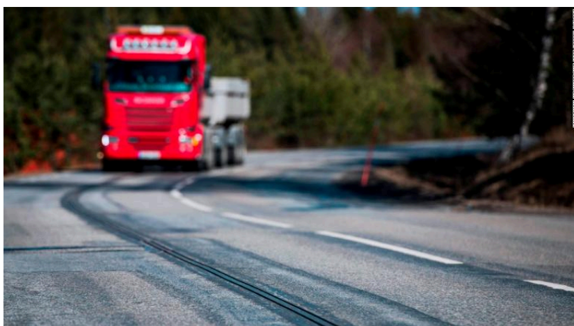
Fig. 1.12 Conductive charging through a power rail in the road, (photo [CNN 2018])
