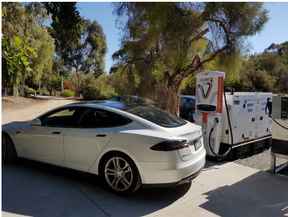
Fig. 6.4 Diesel SAPS powering an off-grid charging DC charging station; (photo courtesy of David Lloyd)
